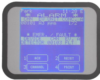
Figure 26) Active Events screen with Alarm and Fault
