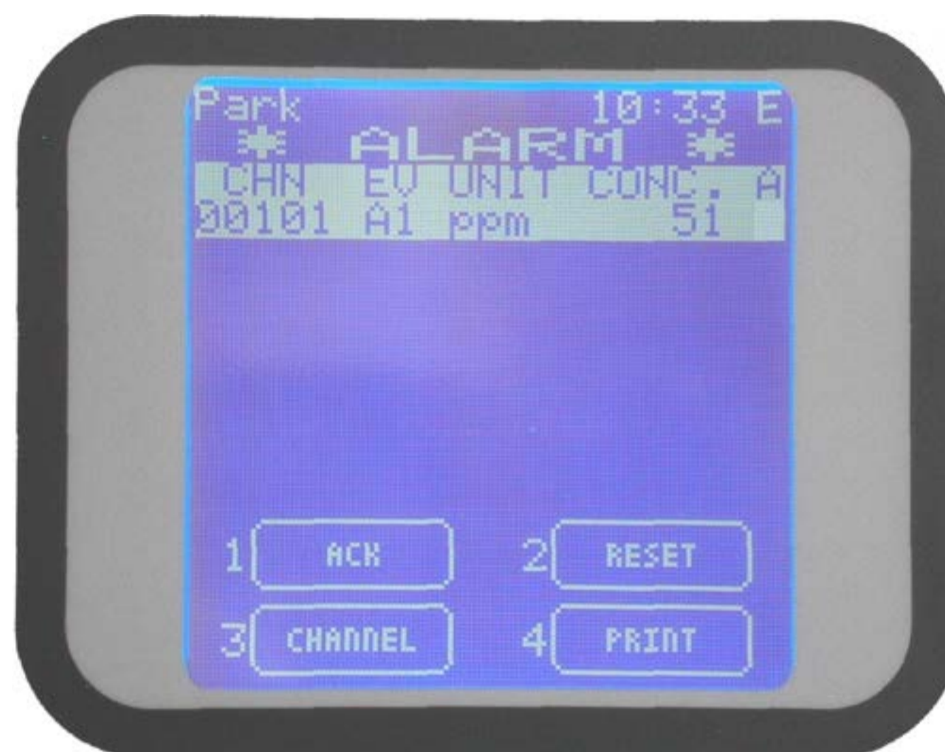
Figure 21 Typical ALARM state of the ACTIVE EVENTS screen.
