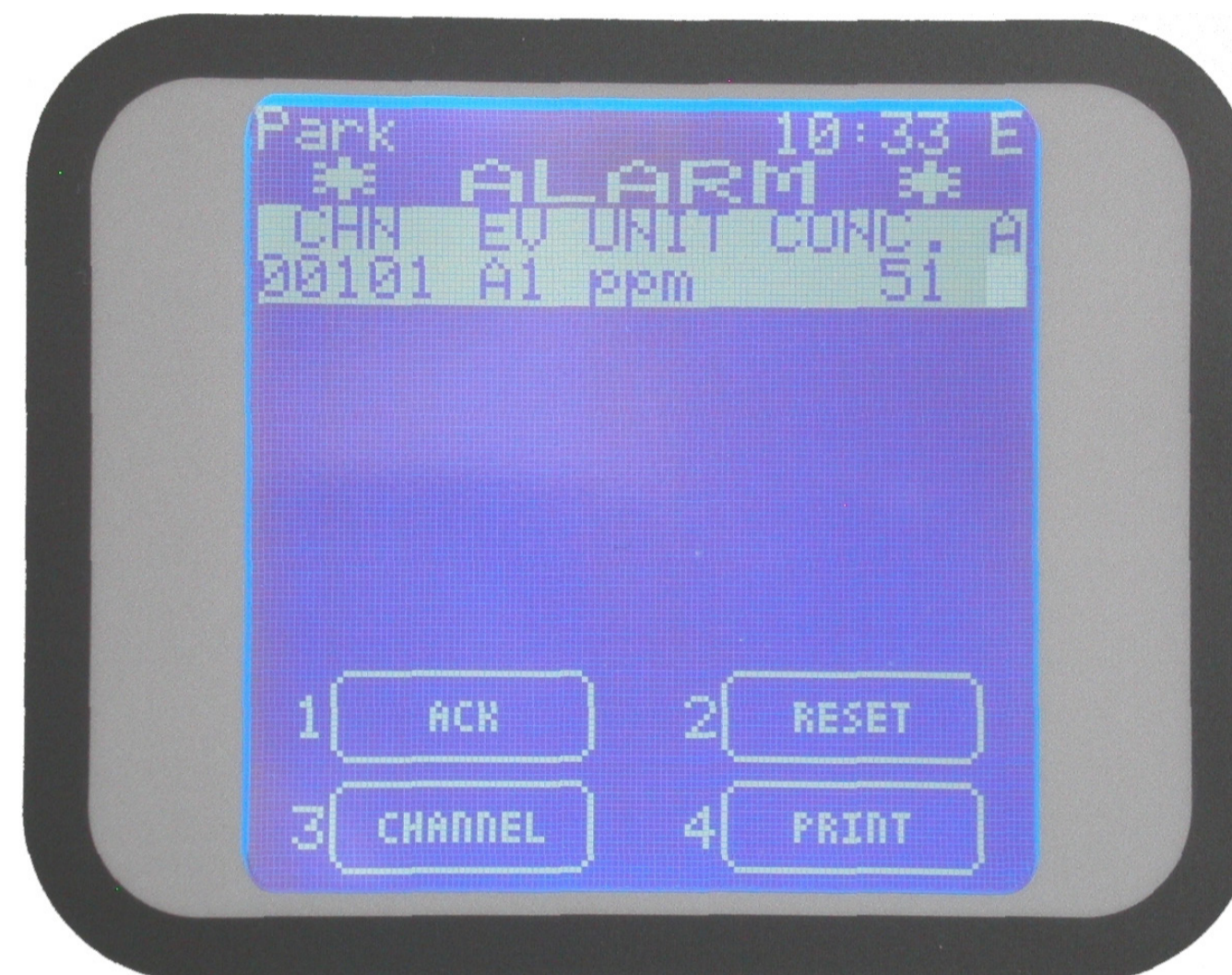
Figure 23 Typical ALARM state of the ACTIVE EVENTS screen.
