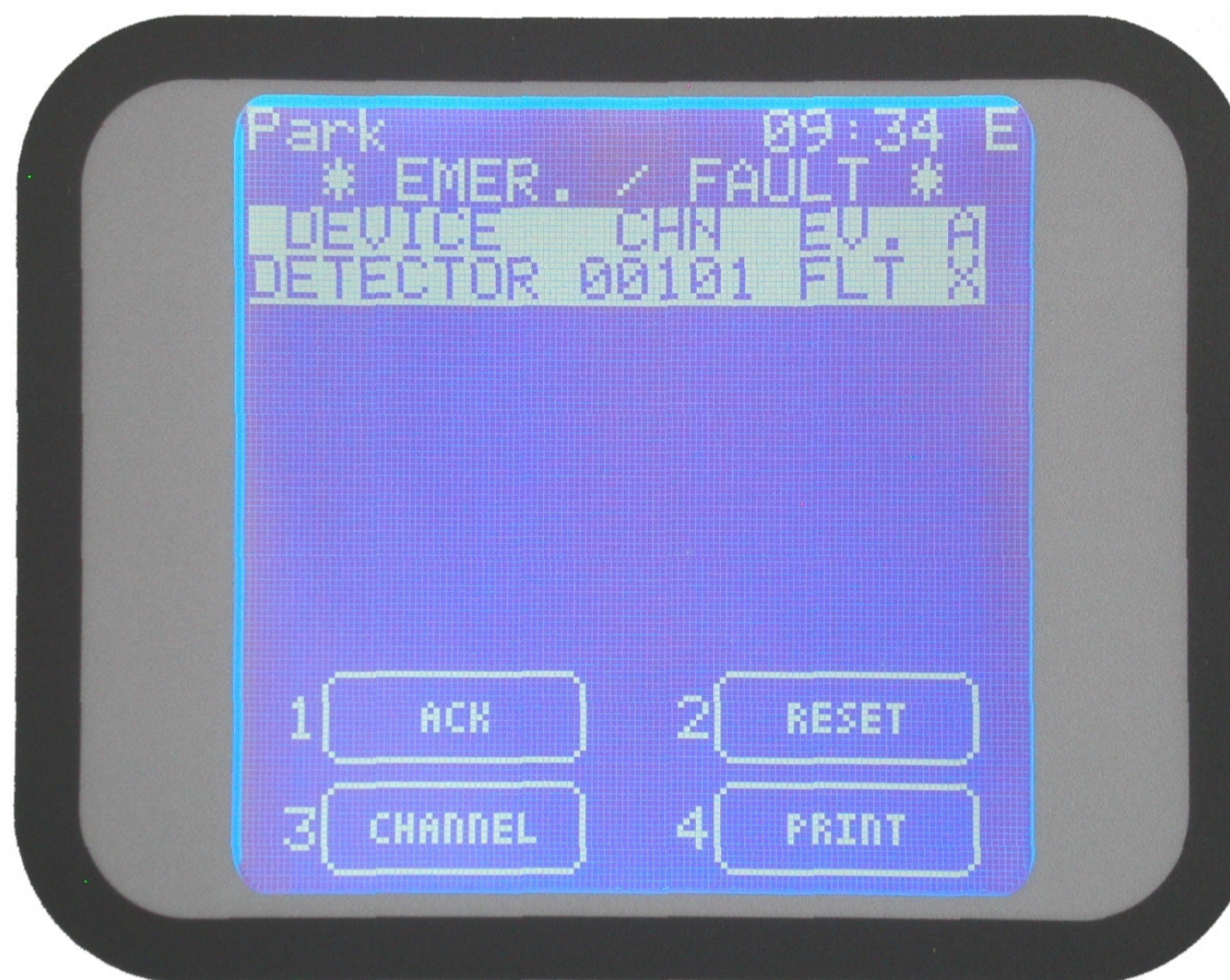
Figure 25 Typical FAULT state of the ACTIVE EVENTS screen.
