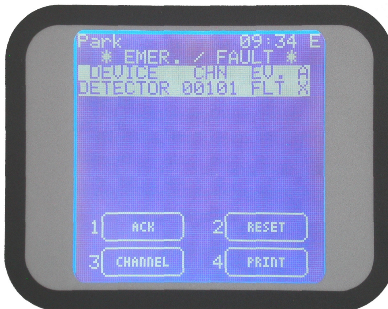
Figure 30 Active events screen with fault only
